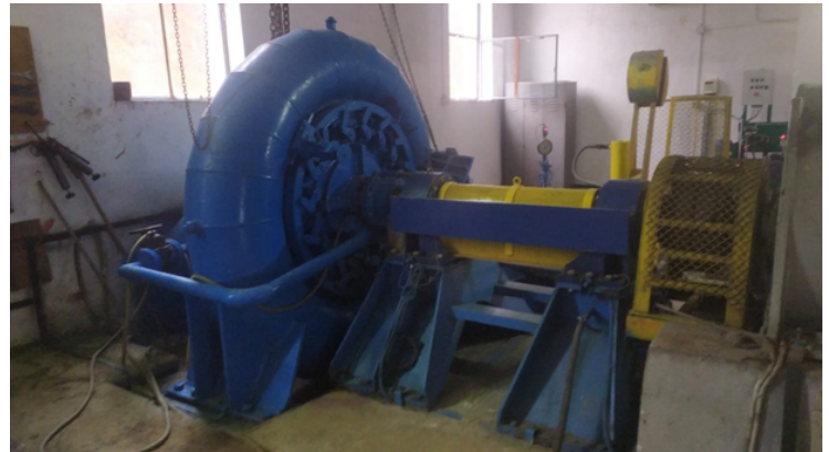
Micro-hydroelectric power plant on the river Barnar. General view of the main building and Francis turbine details.
